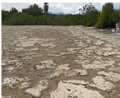
Figure 12k: Cracked grounds becoming visible in parts of Nadi as reported on the 24 th . Source: FBC News.
