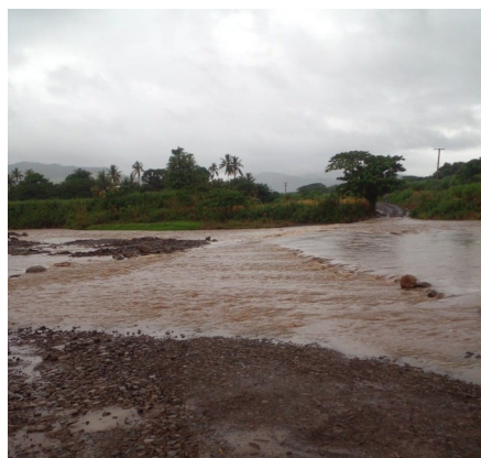
Figure 12h: Toge Crossing, Ba, Western Division, on the 18 th . Source: Fiji Roads Authority.
