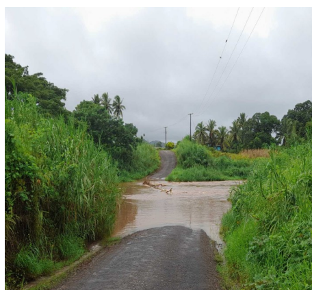
Figure 12d: Nakama Crossing, Labasa, Northern Division, on the 2 nd . Source: Fiji Roads Authority.
