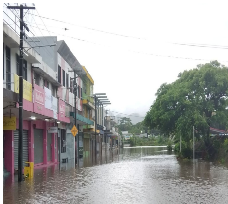
Figure 12a: Rakiraki Town, Western Division, on the 1 st . Source: Fiji Roads Authority.
