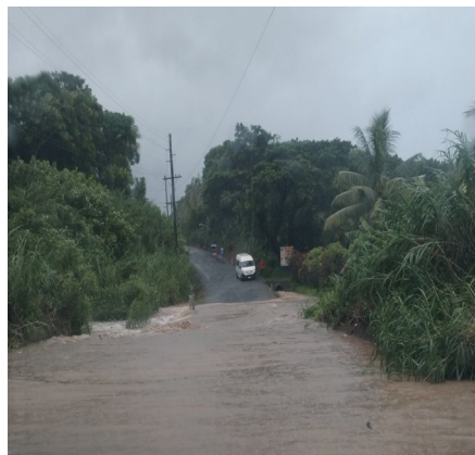
Figure 12b: Naboutini, Central Division, on the 1 st . Source: Fiji Roads Authority.
