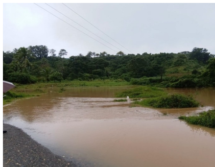
Figure 12b: Inundated Viria Road, Naitasiri Central Division, on the 16 th . Source: Fiji Roads Authority.
