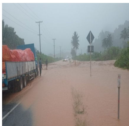
Figure 12d: Inundated Queens road, Vunaniu Flats, Central Division, on the 21 st . Source: Fiji Roads Authority.
