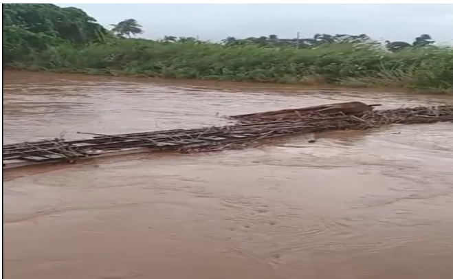
Figure 14p: High waters at a bridge outside of Nadi Town, Western Division. Source: Viliame Nawaqa.
