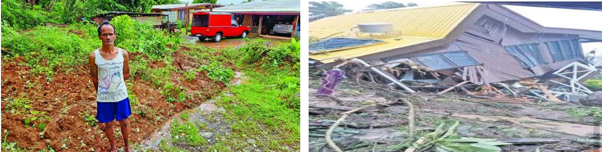
Figure 20: (a) Pile of vegetation, debris and soil materials brought by the landslide at Vunika, Labasa on January 11 th (Picture Credit: Fiji Sun); (b) Damaged house at Nananu-i-Ra due to landslide on January 11 th (Picture Credit: The Fiji Times).
