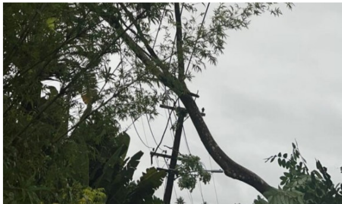
Figure 12b: Trees falling over the power pole in Tamavua due to the landslide on 3 rd June, 2023. Source: FBC News
