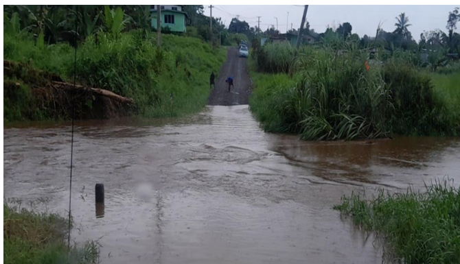
Figure 12k: Waisa Bridge on the 21 st . Source: National Disaster Management Office.
