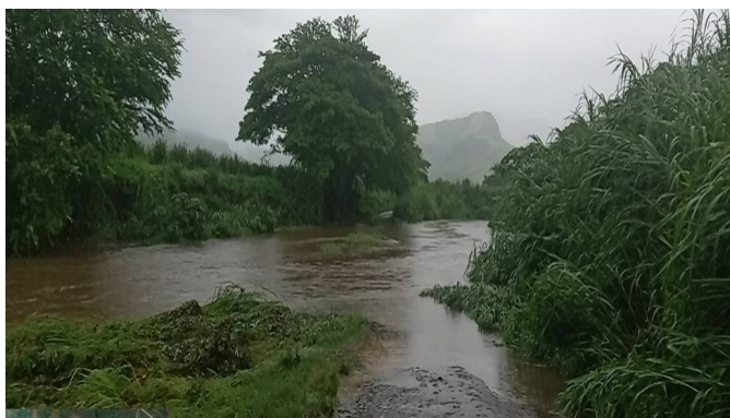
Figure 12q: Katudrau Crossing, Rakiraki on the 25 th . Source: Fiji Roads Authority.
