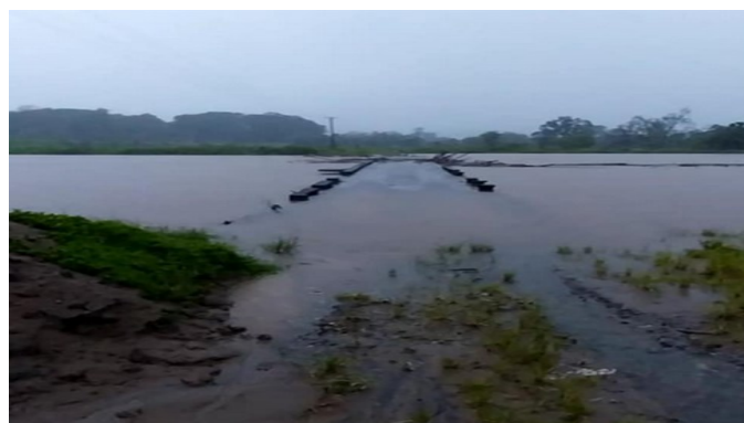
Figure 12e: Old Naqali Bridge on the 16 th . Source: National Disaster Management Office.
