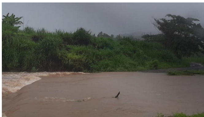
Figure 12r: Marinitawa Road, Ba on the 25 th . Source: Fiji Roads Authority.
