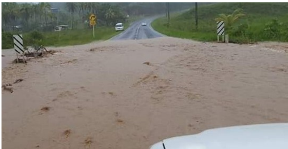
Figure 17: Flooded Vunaniu flat on the 16 th . Picture source: Fiji Government.
