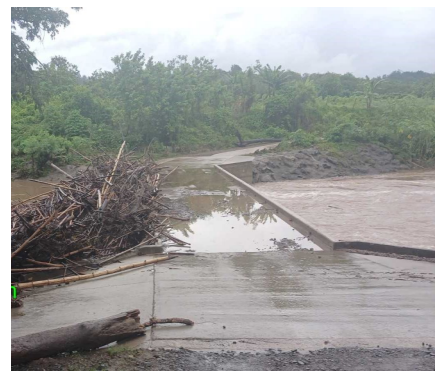
Figure 12c: Flooding and blockage of Emuri crossing, Nadroga, on the 25 th . Source: Fiji Roads Authority.
